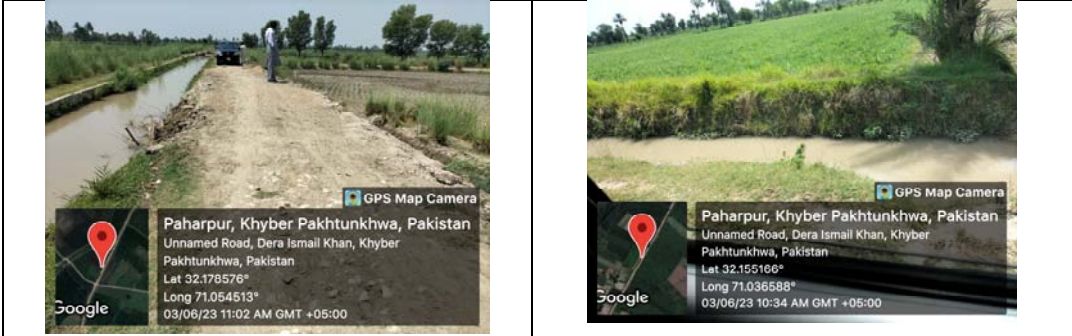
Rehabilitation of damaged/washed away Canal Section of Kat Garh Minor
