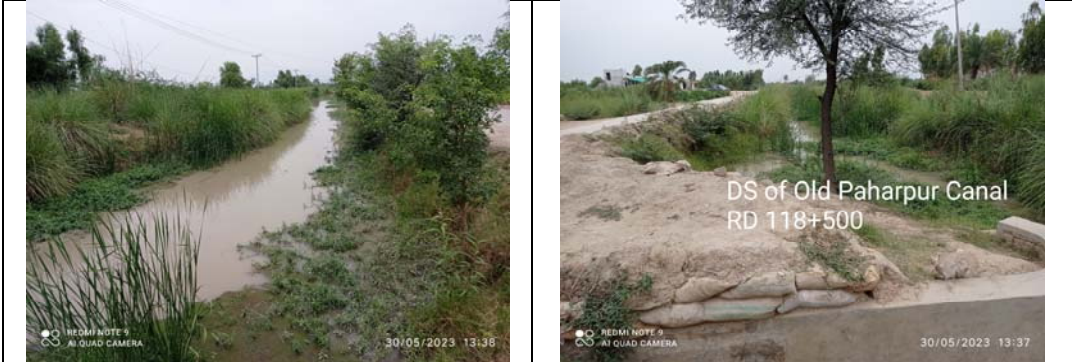
Rehabilitation of damaged/washed away Canal Section of Old Paharpur canal (RD. 118+500-122+300)
