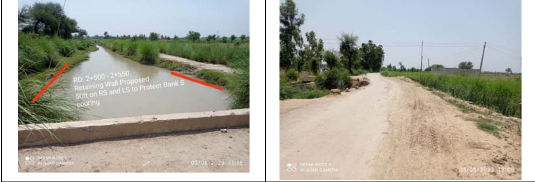
Rehabilitation of damaged/washed away Canal Section of Girsal Feeder
