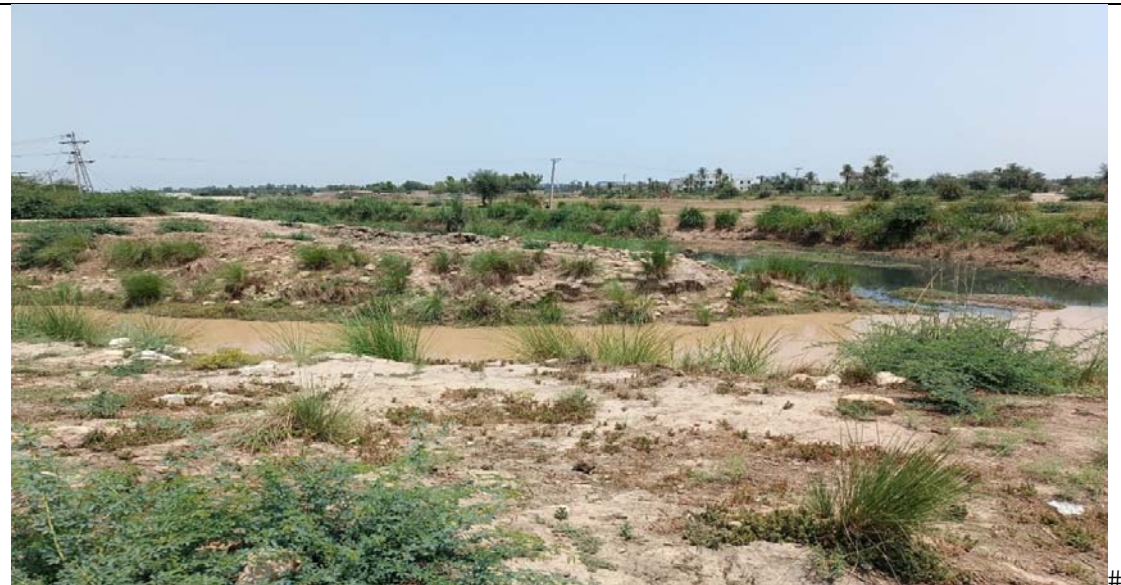
Proposed Stone Pitching at Confluence of Two (02) Drains
